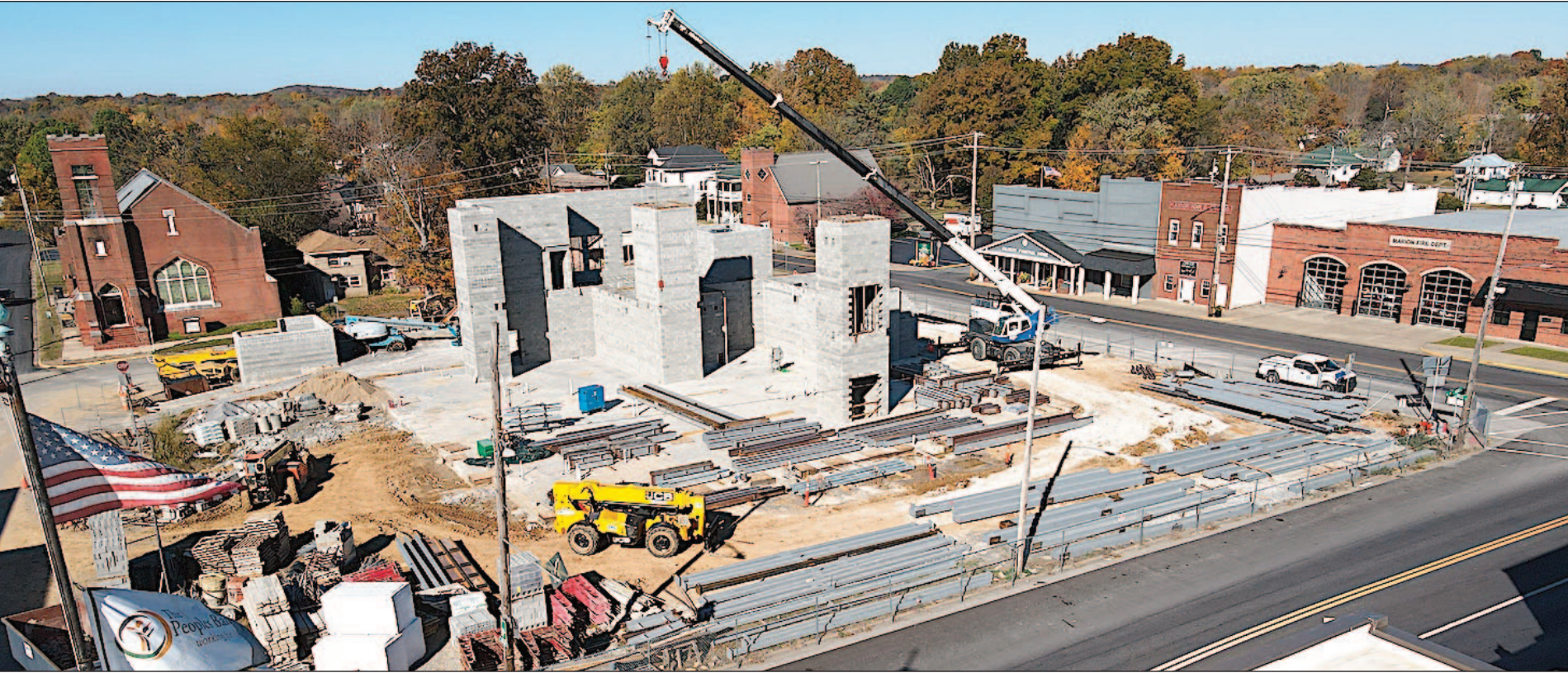
Taking Shape It will be another 18 months before the new courthouse will be ready to occupy, but construction is picking up steam in downtown Marion with the arrival of a large crane last week. If you drive by it every day, perhaps the subtle changes are not as noticable, but work is proceeding on schedule thanks to fortuitous fall weather. Pinnacle Inc., of Benton is the general contractor. A live video link to see what's happeneng daily is available at The-Press.com.
