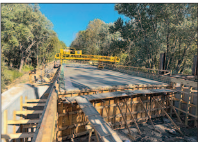
Decking was recently poured on part of the Dam 50 bridge.
